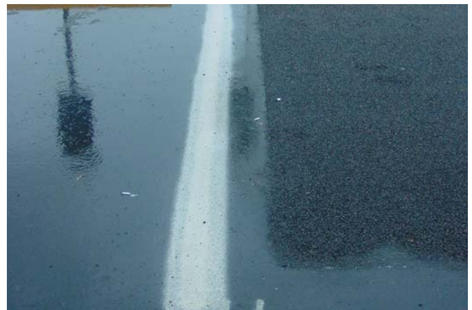
Fig. 1.8 A comparison of traditional asphalt (left) and porous asphalt (right) when wet. The gaps created by leaving out the finer particles in porous asphalt allow water to infiltrate pavement and into a gravel reservoir below. As a result, porous asphalt appears dull when wet, because the water runs through and does not pond, also creating a high friction surface.
