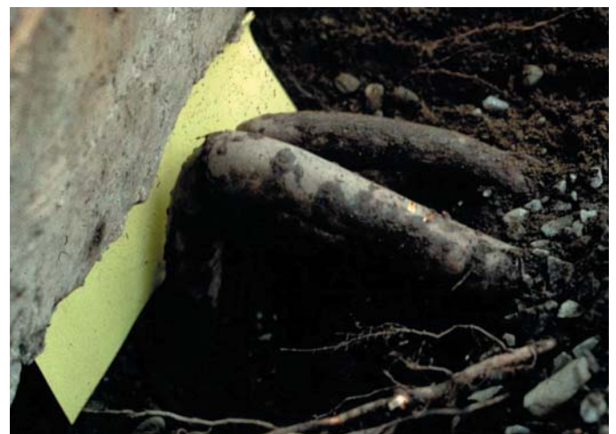
Fig. 1.19 Roots near pavement adapt and change direction when they hit the side of the paving profile.
