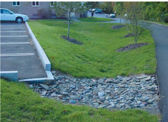
Fig. 1.3 Example of a retention/detention pond adjacent to a surface lot at Cornell University, Ithaca, NY. This treatment uses space that could be otherwise directed towards other uses.
