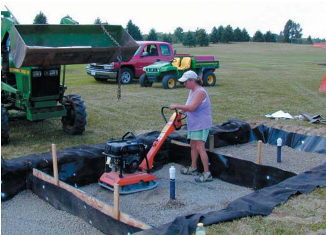
Fig.1.13 Compaction of CU-Structural Soil® in a test plot on the Cornell University campus. A vibrating tamper compacts CU-Soil™ so that pavement may be laid on top.
