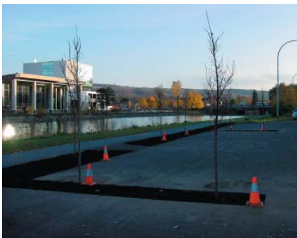
Fig 1.32 Research Parking Lot in Ithaca, N.Y. The foresection is traditional asphalt on CU-Structural Soil® while the back section of the lot is constructed of porous asphalt on CU- Structural Soil®.
