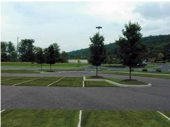
Figure 13. Photo simulation of turf-covered perimeter parking at a big box lot in Ithaca, NY. For best results, turf should be only placed in parking stalls and not in driving lanes of the parking lot.
