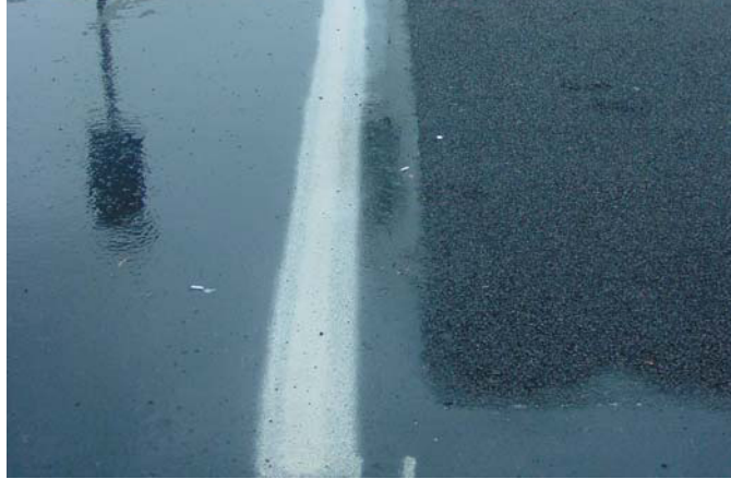
Figure 18. A comparison of traditional asphalt (left) and porous asphalt (right) when wet. The gaps created by leaving out the finer particles in porous asphalt allow water to infiltrate pavement and into the structural soil reservoir below. As a result, porous asphalt appears dull when wet, because water runs through and does not pond, which creates a high friction surface.
