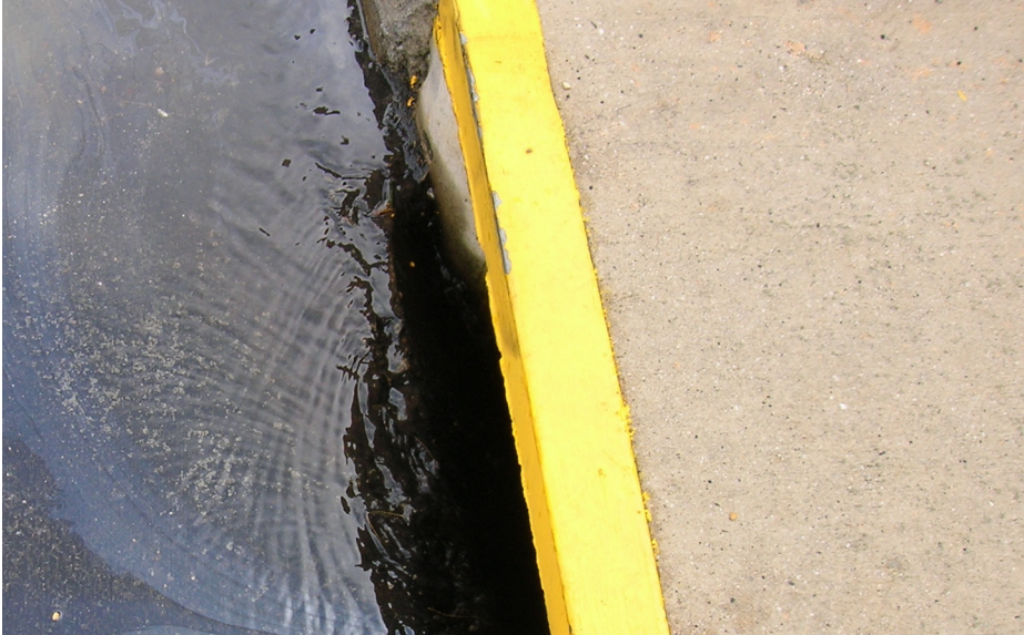
Figure 1. Typical runoff from a parking lot going into a storm sewer. Notice that traces of oil are visible to the naked eye. There are many other pollutants in parking lot runoff such as various metals, sediment, salts, and litter.
