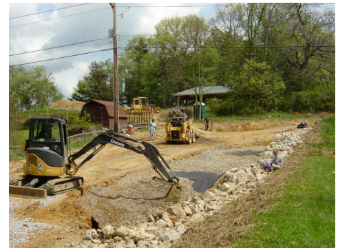
Figure 8. The top illustration shows a diversion mound system as used on a roadway. The photo to the left shows the installation of diversion mounds for an access road. The diversion mounds are circled in red. In the photo to the right you can see the mounds during the structural soil installation process.
