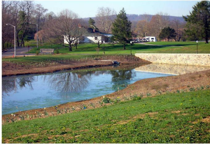
Figure 3. An example of a retention/detention pond adjacent to a conference center on the Virginia Tech campus in Blacksburg, Virginia. This treatment uses space that could be otherwise directed towards other uses.
