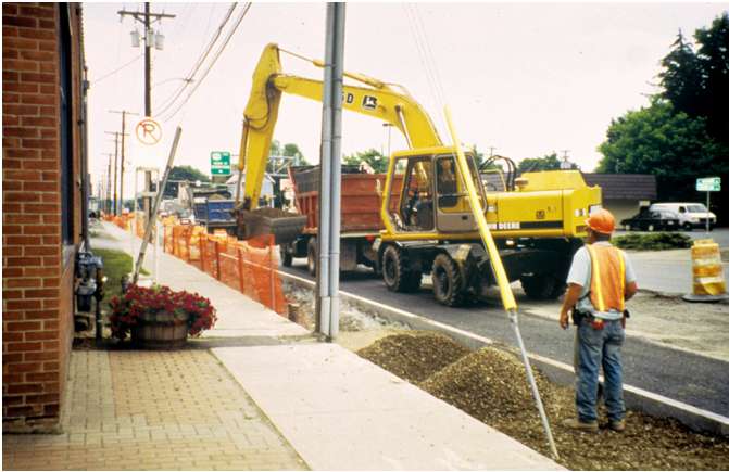
Fig.1.9 Installing CU-Structural Soil™ in Ithaca, NY in 1997
