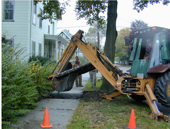
Fig. 1.20 Break-out zone with CU-Structural Soil™ under a sidewalk between a narrow tree lawn and adjacent landscape area
